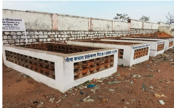
Compost Facility Jatara (Tikamgarh)
