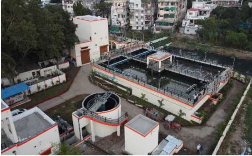
5 MLD STP AT SHIRIN RIVER
