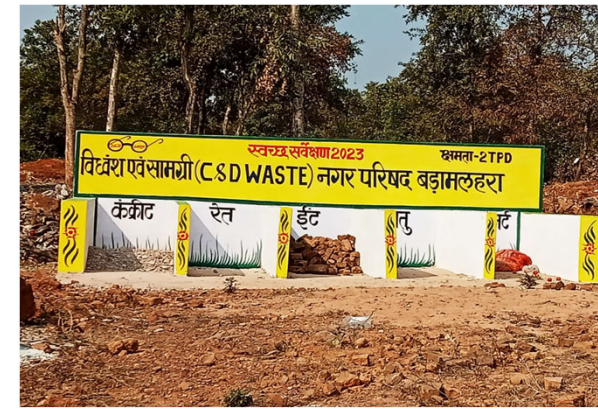
C&D Collection Facility Bada Malhera (Chhatarpur)
