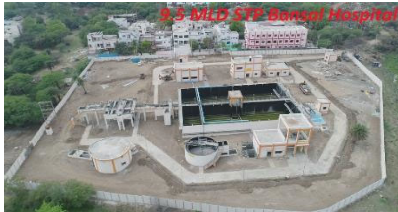
9.5 MLD STP AT BANSAL HOSPITAL
