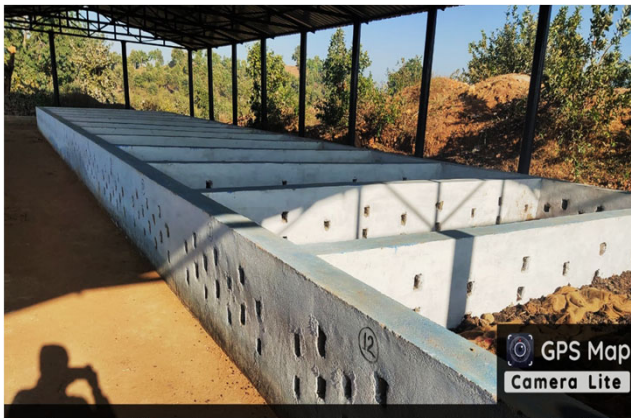
Composting Facility Umariya (Umariya)
