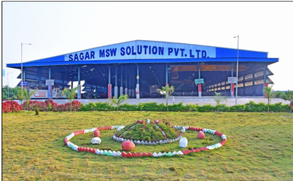
Sagar Cluster Integrated MSW Processing Plant
