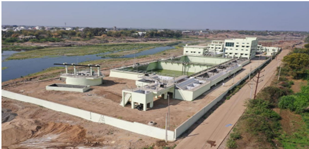
17.6 MLD STP IN KHARGONE
